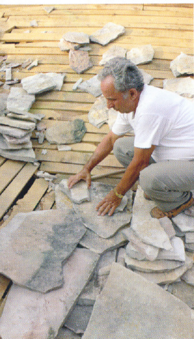
A roof builder at work
