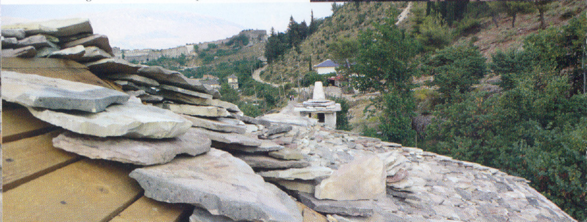
Roof tiles waiting to be hammered into place
